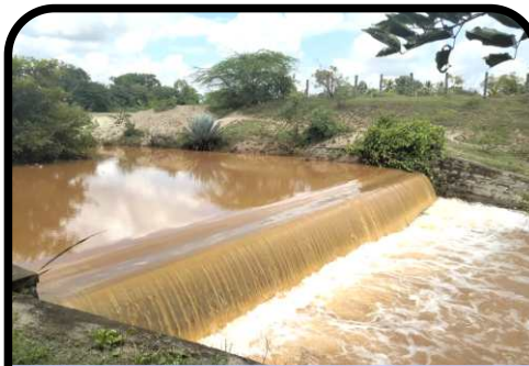
Check Dams overflowing at Kellamballi
