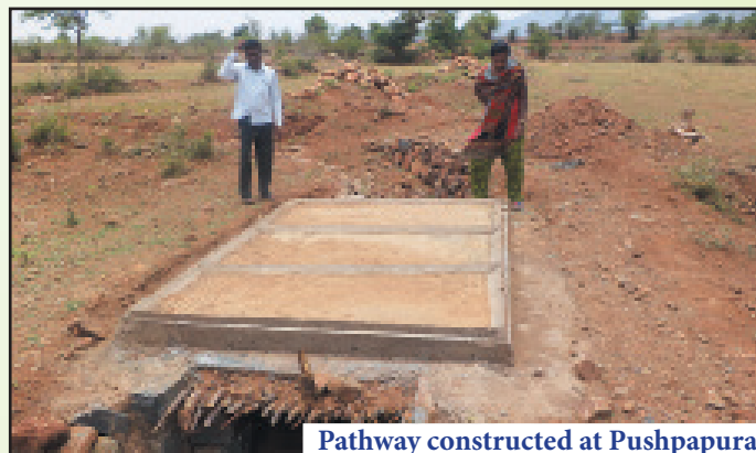
Pathway construction work
