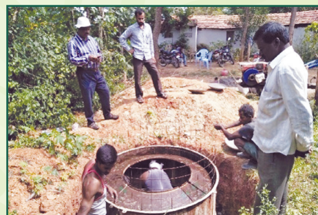
Construction of Bio-Gas
