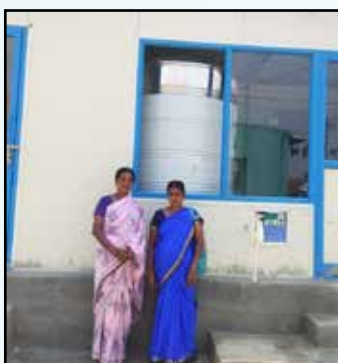
Drinking water unit
