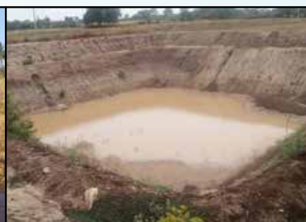
Rain water conserved in Farm pond
