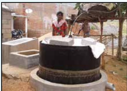
Construction of bio gas plant
